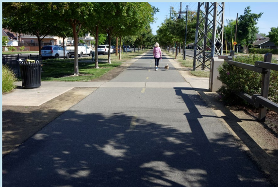
Class I: Completely separated right of way for bicycles and pedestrians, such as a paved multi-use trail
