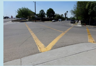
Sloped intersection along Belmont Avenue
