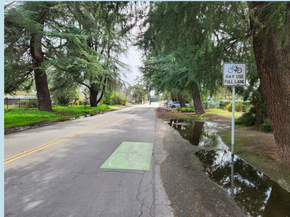
Class III: Shared on-street facility for bicycles and vehicles, marked with signage
