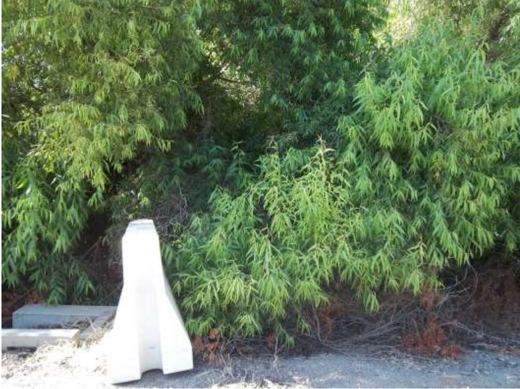
West end of bridge looking south
