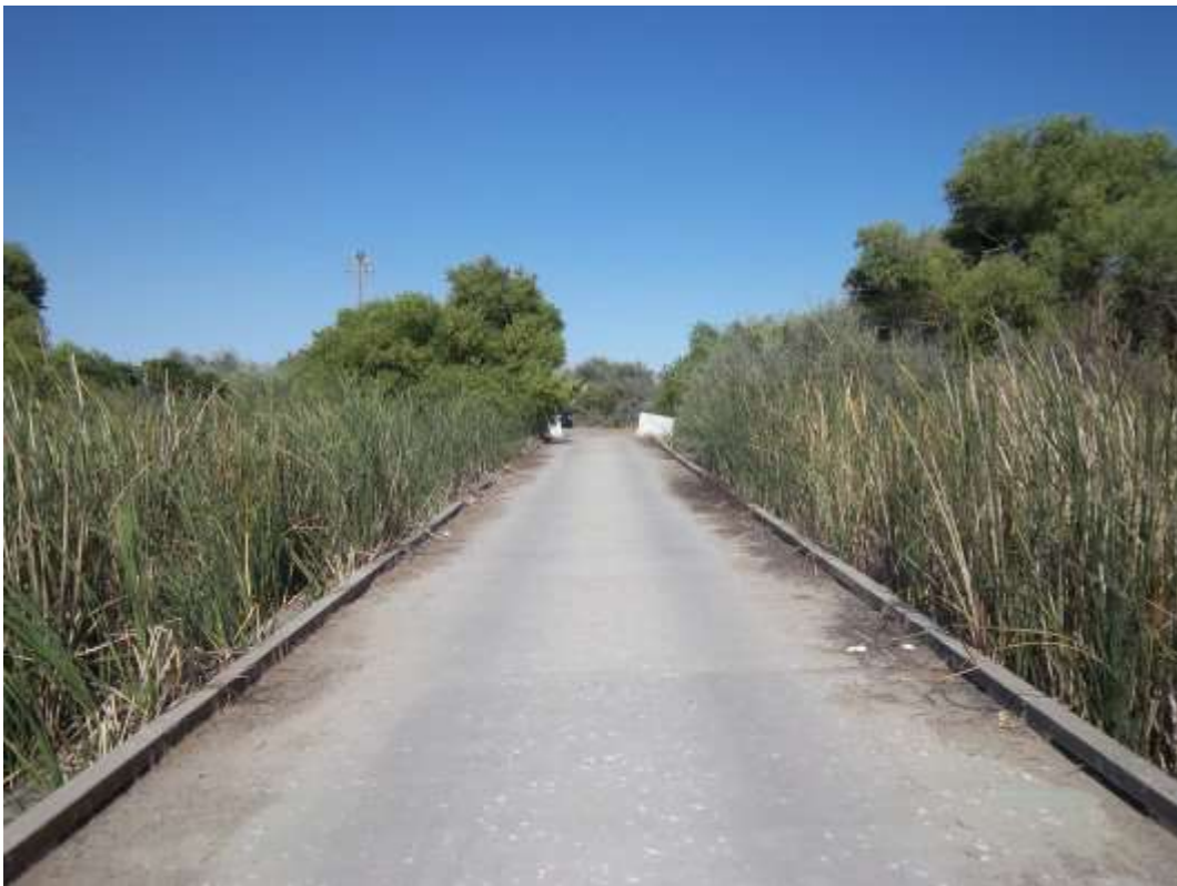
Middle of bridge looking west
