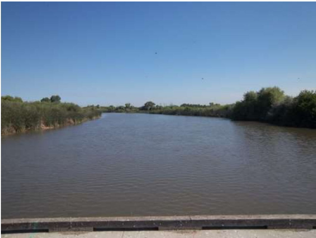
Middle of bridge looking downstream
