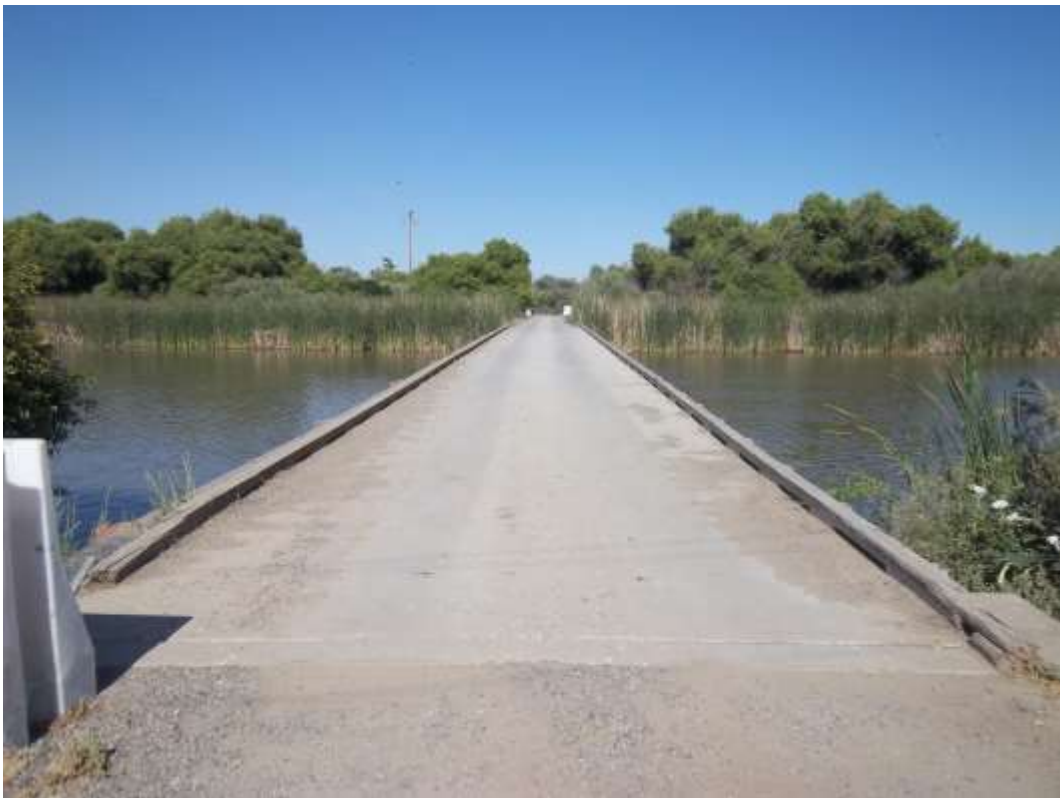
East end of bridge looking west
