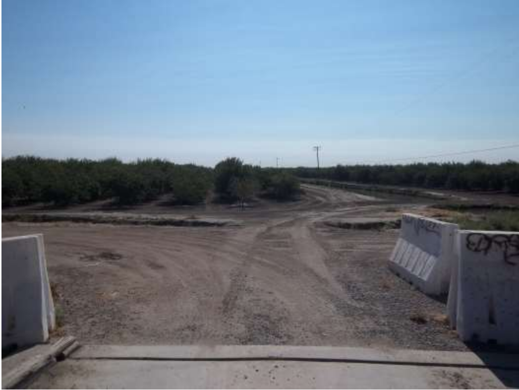
East end of bridge looking east
