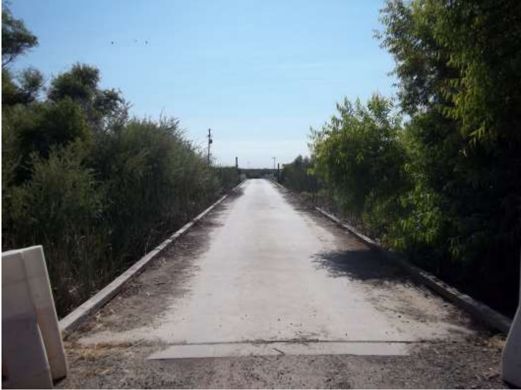
West end of bridge looking east
