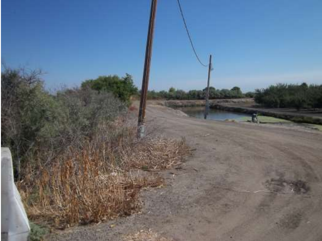
East end of bridge looking north
