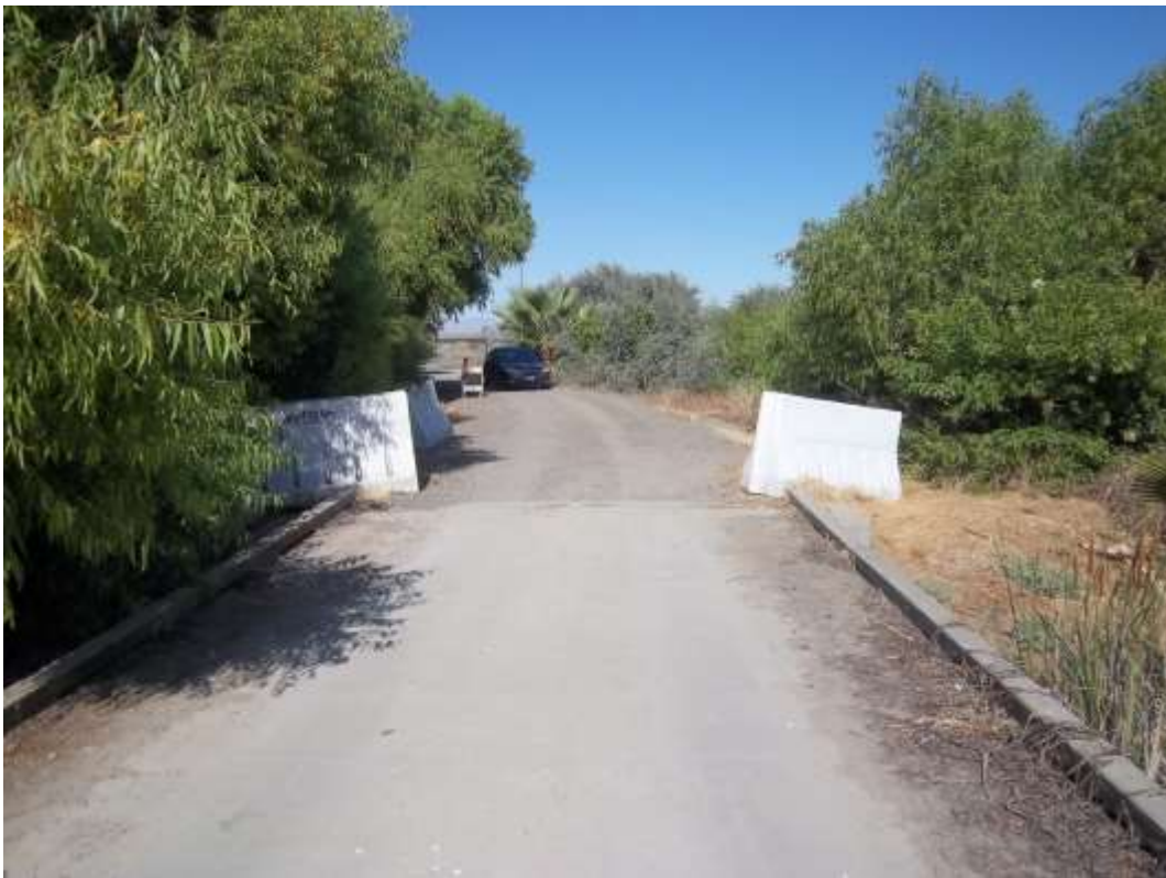
West end of bridge looking west
