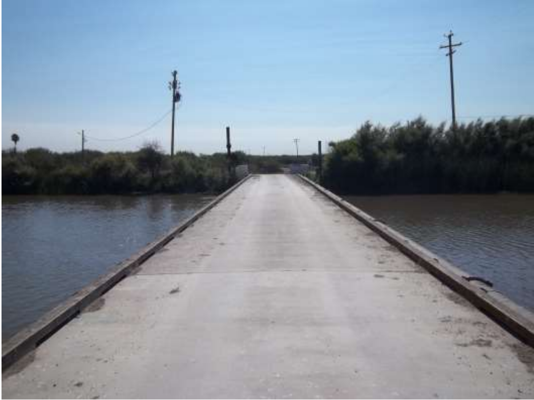
Middle of bridge looking east
