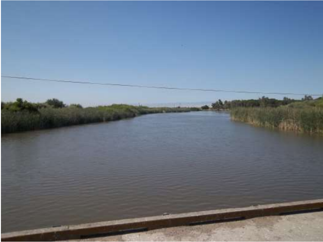
Middle of bridge looking upstream
