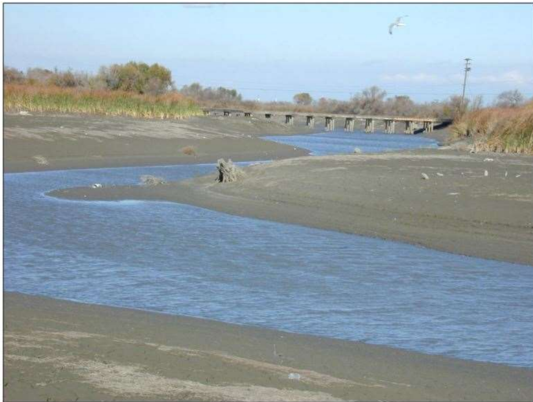
Figure 3-2. Existing Bridge, Circa 1999
