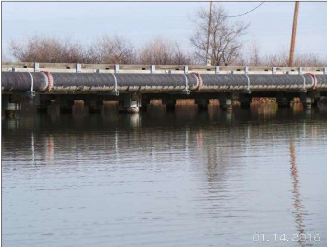
Figure 3-5. Existing 20-inch Water Line on Bridge
