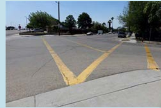
Sloped intersection along Belmont Avenue
