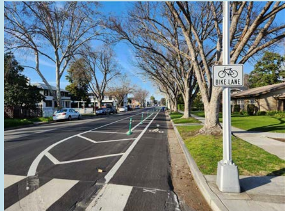
Class IV: Physically separated bicycle facilities that are distinct from the sidewalk, such as an on-street bike lane separated from vehicle lanes by bollards or street parking
