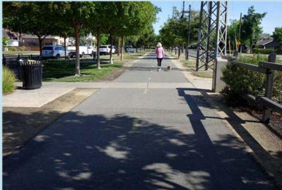
Class I: Completely separated right of way for bicycles and pedestrians, such as a paved multi-use trail
