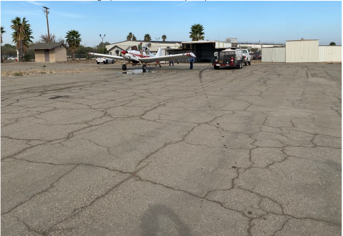
Photograph 6 – The current Apron pavement condition.
