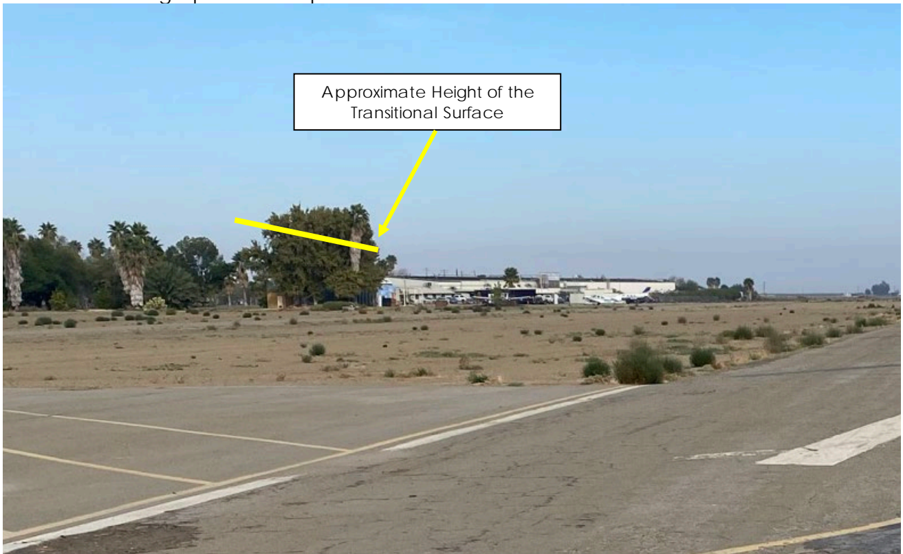
Photograph 7 – Trees penetrate the CFR Part 77 Transitional Surface.
