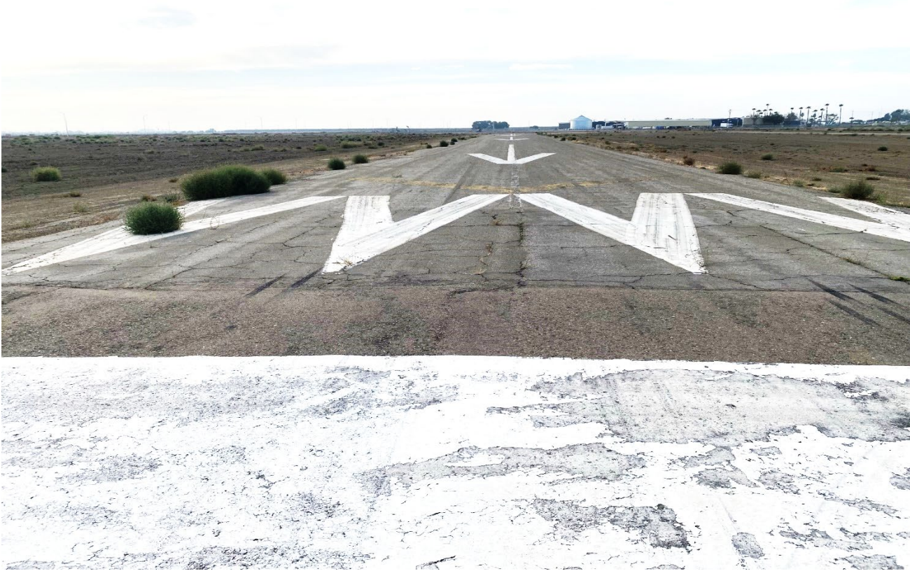
Photograph 1 – Example of the current Runway pavement condition.
