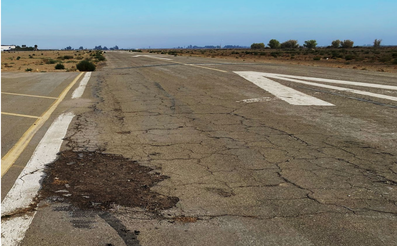
Photograph 3 - Example of the current Runway pavement condition.
