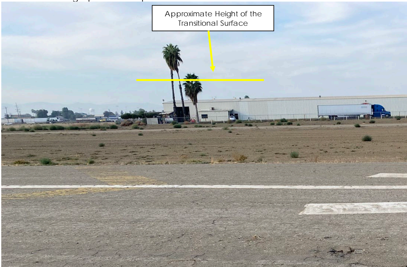
Photograph 8 – Trees penetrate the CFR Part 77 Transitional Surface.
