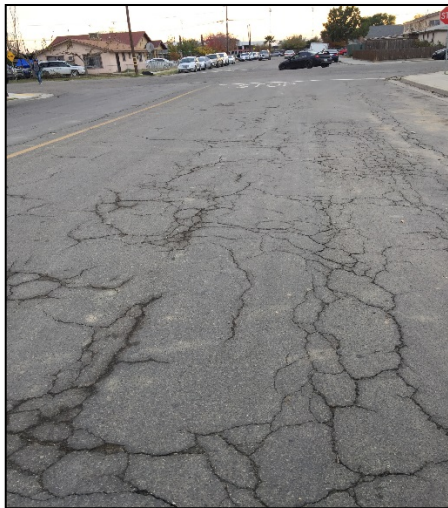
PCI = 40 (Poor)
